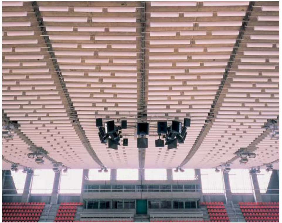
illbruck rondo absorber, St. Jacob Sports Facility, Basil, Switzerland
