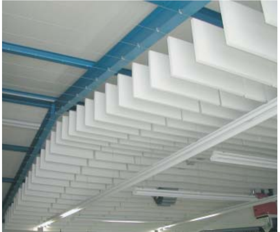
illbruck plano absorber ECO, KTD, Calw, Germany
